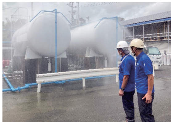
Emergency response training for fire extinguishing
